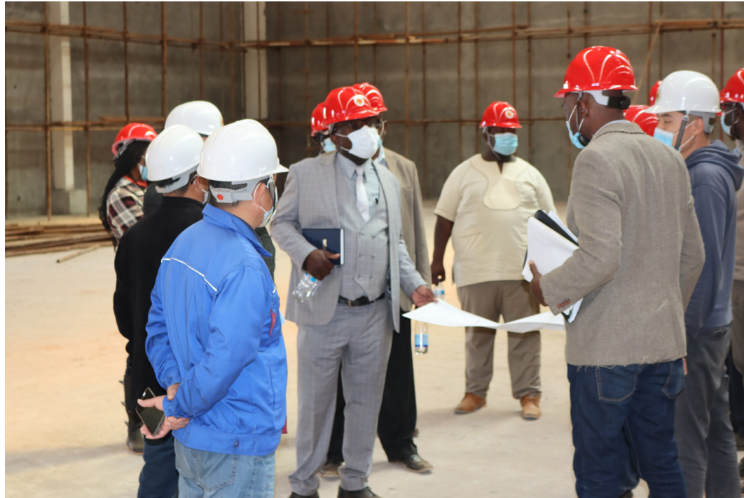
Chinese contractors shows NatPharm Internal Audit Manager, Mr Brain Mutseyami (left) and Mutare Branch Manager, Mr Kudakwashe Chimbarara (partly obscured) the new warehouse plan
